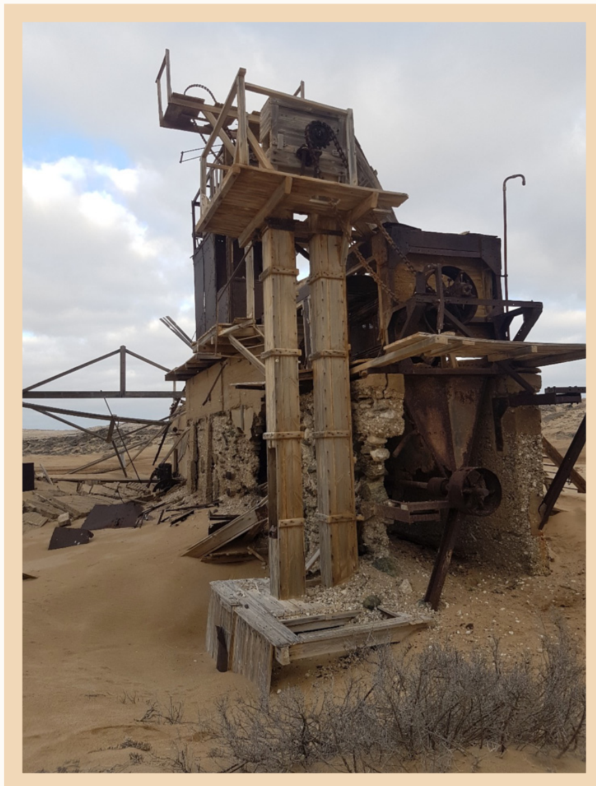
Figure 87 Diamond ore processing plant at Charlottental
