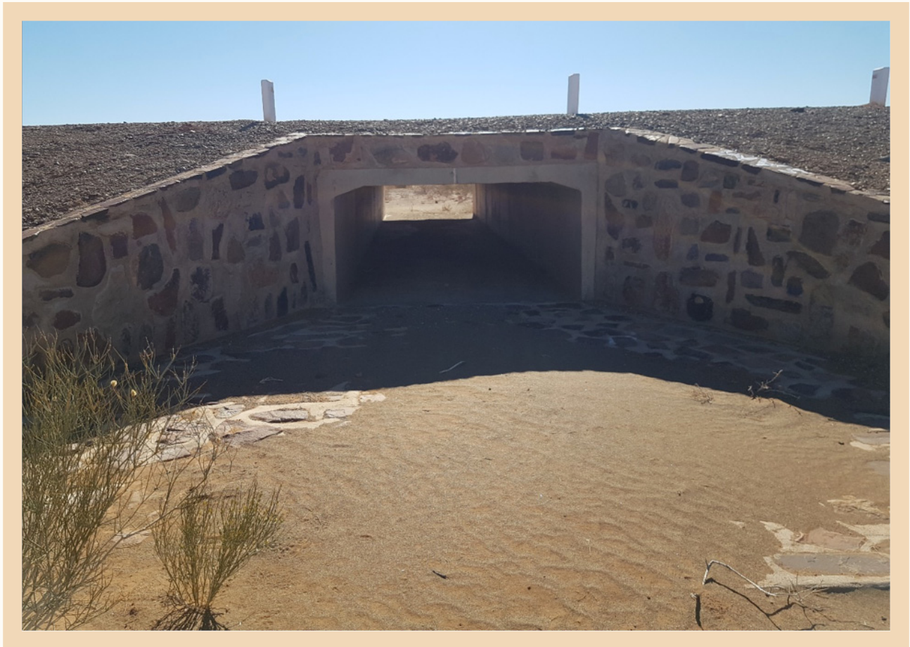
Figure 29 Large culvert under the Aus-Rosh Pinah Road
